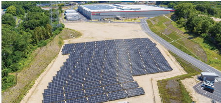
Establishment of photovoltaic power generation facilities (1,134 kW at Seto Factory)
