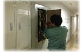
Communication facility construction
