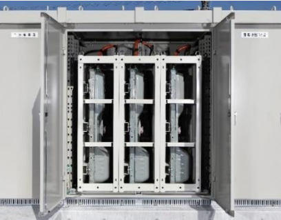
Storage battery equipped with an EV reused battery pack
