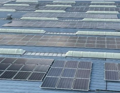
PV reused panel (5 different specifications)
