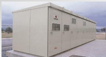
High-voltage power receiving equipment
