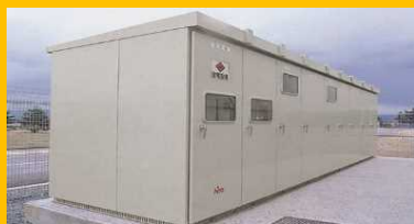
High-voltage power receiving equipment
