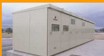
High-voltage power receiving equipment
