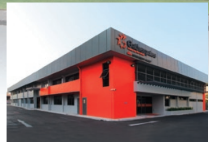
●Gathergates Group Pte Ltd Republic of Singapore (Head office) Malaysia (Plant) [Business scope] Manufacture and sales of electrical and mechanical equipments such as panel boards, control panels, and meter boxes.
