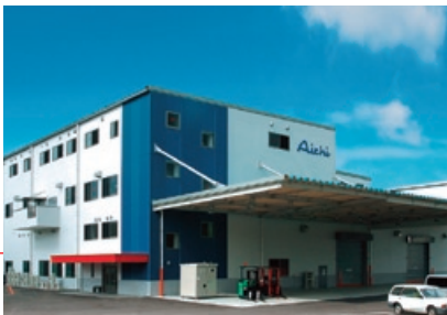
●AICHI ELECTRIC WORKS CO., LTD. Komaki City, Aichi Prefecture [Business scope] Design, manufacture, sale, and repair of mechanical equipments for electricity.
