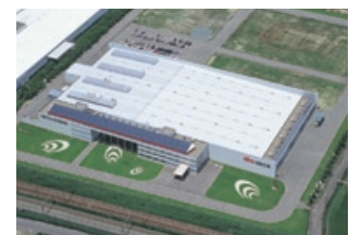
●Kakegawa Plant Kakegawa City, Shizuoka Prefecture [Land] 68,000m 2 [Buildings] 16,000m 2 [Main products] Compact enclosures
