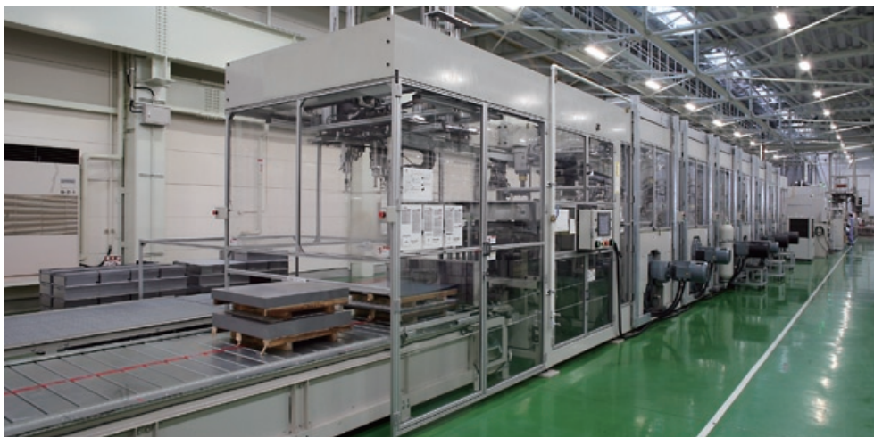
Kakegawa plant [Production line of CH type Enclosures]
