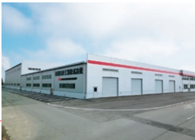
●TOHOKU NITTO KOGYO CORPORATION Hanamaki City, Iwate Prefecture [Business scope] Manufacture of electric and mechanical equipments and components
