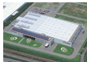
●Kakegawa Plant Kakegawa City, Shizuoka Prefecture [Land] 68,000m 2 [Buildings] 16,000m 2 [Main products] Compact enclosures
