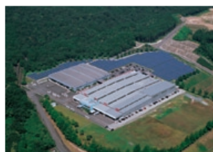
●Karatsu Plant Karatsu City, Saga Prefecture [Land] 100,000m 2 [Buildings] 16,000m 2 [Main products] High-voltage power receiving equipment, Panel boards
